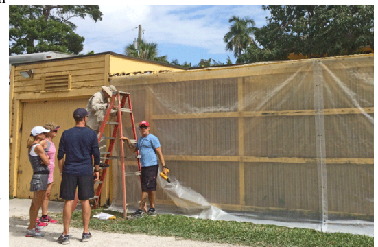
FLOS members Craig Barry and Richard Mach installing the winterizing panel on the west wall of the Lath House at Bonnet House
